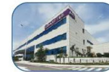
Qingdao Sino-German factory (Electric water heater)
